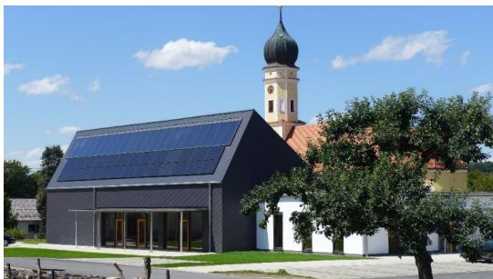
Photovoltaikanlage in Oberhausen
