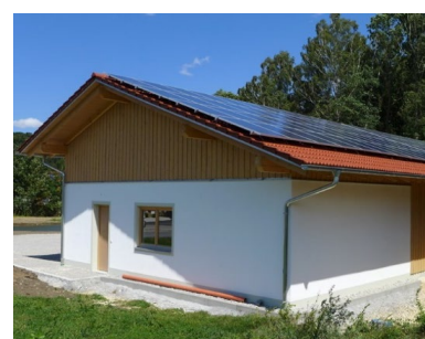
Photovoltaikanlage in Oberhausen
